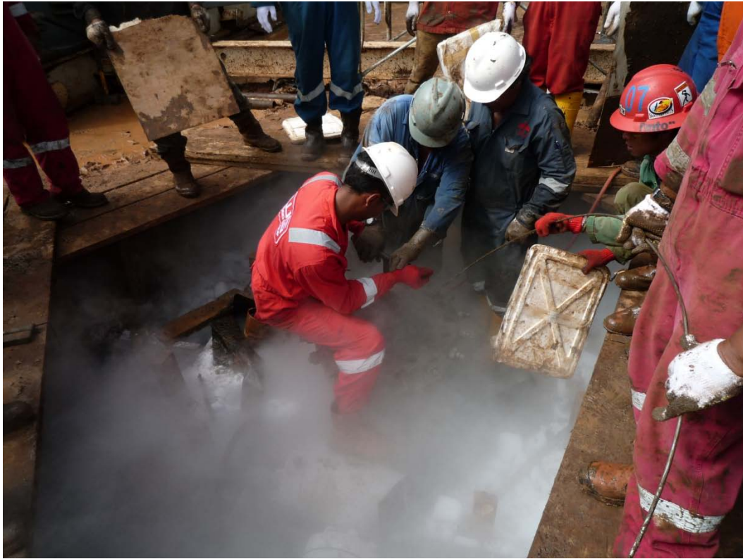
Installation of the BPV in tubing hanger (second barrier installed)
