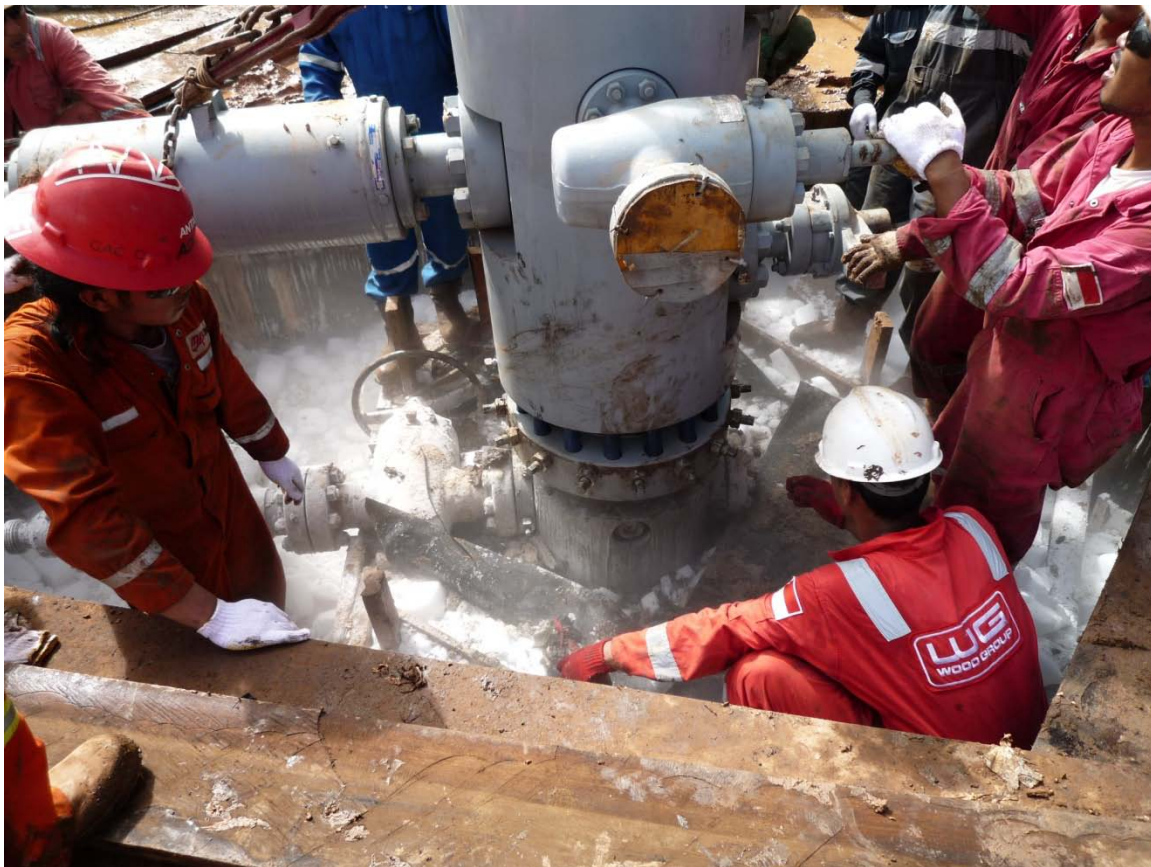
Installation of the tree (well fully secured!)
